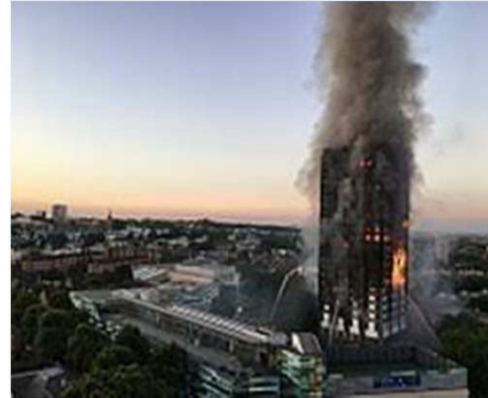
Grenfell Tower Fire – June 2017
